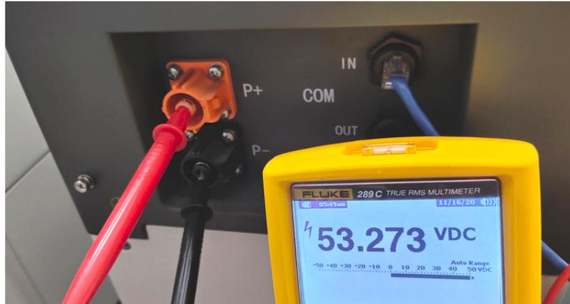
The voltage measured on the PDU is the average voltage of all modules in the tower and should be around 50V. **NOTE: the PDU output voltage will only be correct if the battery has been configured correctly via app and then restarted. Without correct app configuration, the PDU output voltage will be wrong!**
